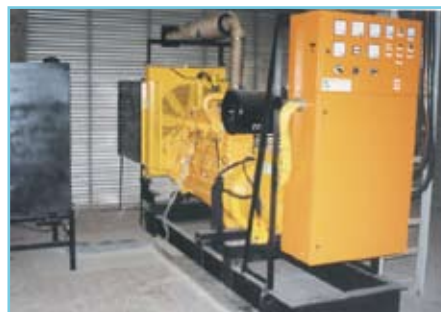
300KVA Automatic mains failure
