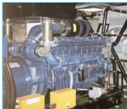
1000KVA Automatic mains failure Generator Set. MTU 16V 2000 G62 / Leroy Somer (Installed at the Capital Alliance Building, Johannesburg)
