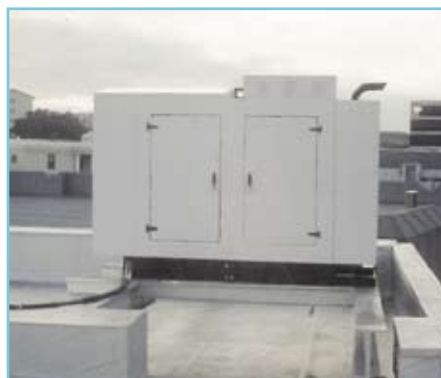
30KVA Automatic mains failure soundproof Generator Set. Standard soundproof canopy with sound levels of 65dB(A) at 7 metres in an open field.
